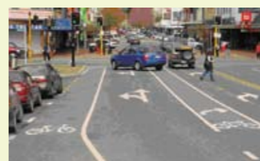
Cycle lanes and advanced stop boxes at Trafalgar Street/Halifax Street signals
